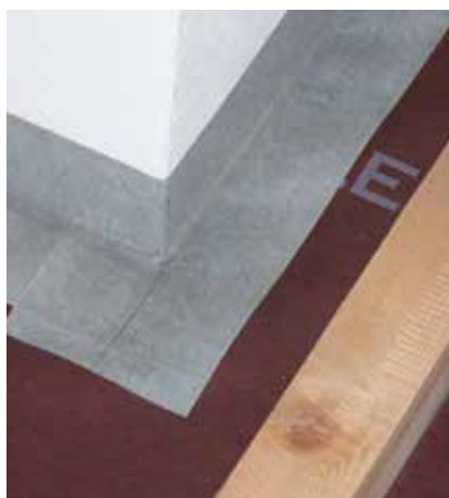
Sealing of a chimney with AIR Coll 150 X with the possibility of plastering over
