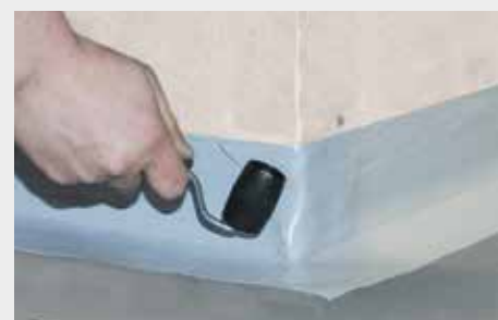
Sealing on plaster and masonry
