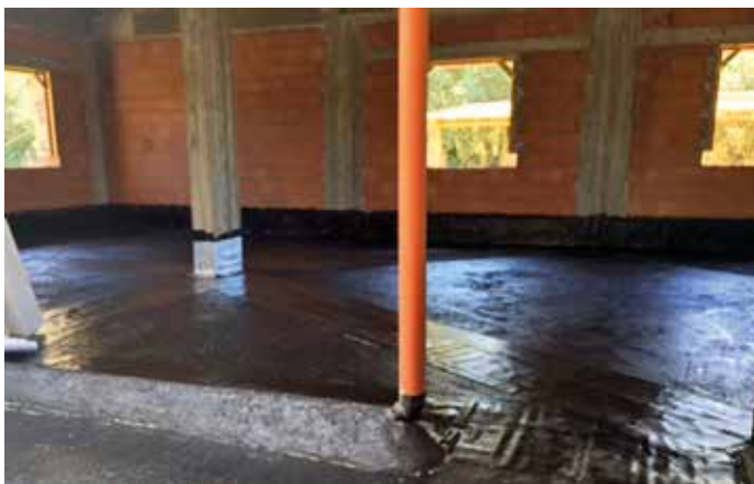
Preparation of the surface using USB Primer BIT
