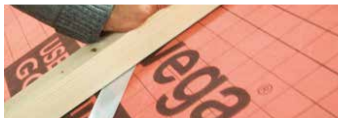
Laying of double adhesive USB Tip KONT DUO with removal of the liner
