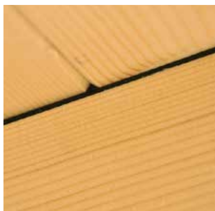
Creating an airtight seal where the matchboard rests on the joist
