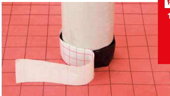
2. Remove the remaining protective liner.
