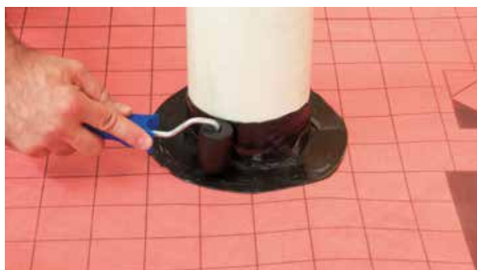
6. Press firmly onto the protuberance with the roller.
