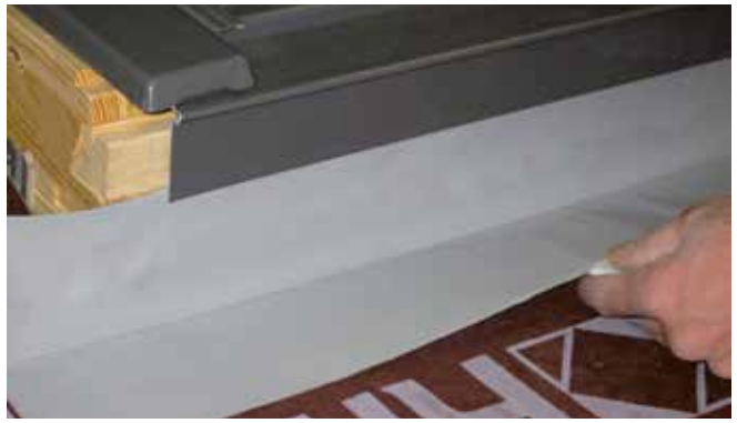
2. Lay USB Coll 150 X tape on bottom part of the window
