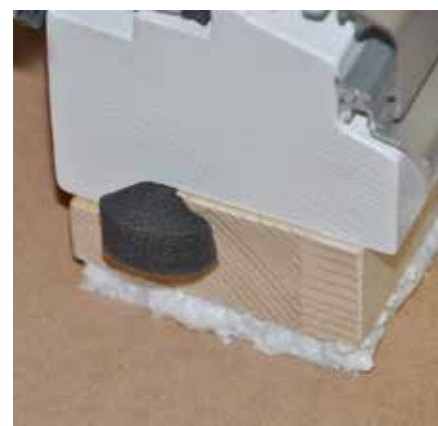
Creating an airtight seal between door or window frame and subframe
