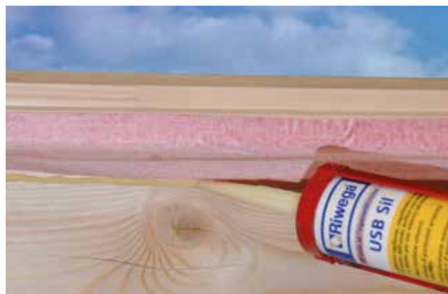
Gluing of internal tape FDB Tape Int AC on wood
