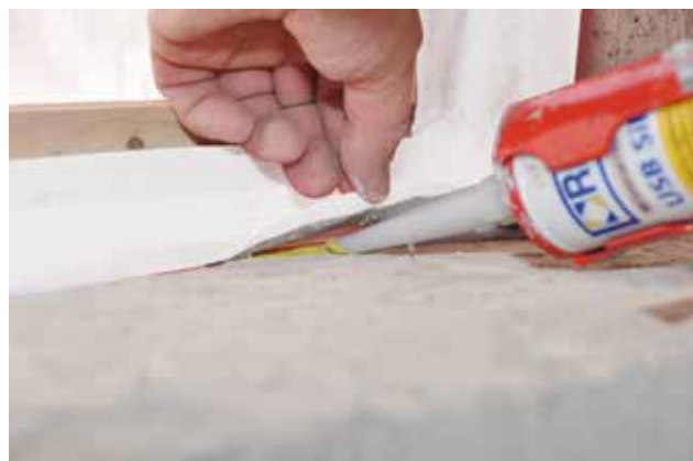
Gluing of external FDB Tape Ext AC tape on masonry
