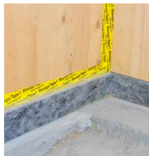
Waterproofing of cill beam
