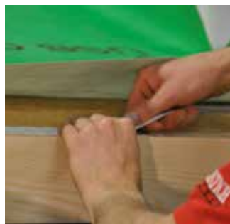
Sealing between membrane and wood
