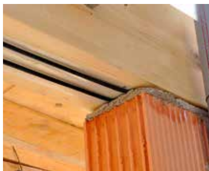
Sealing cill-beam
