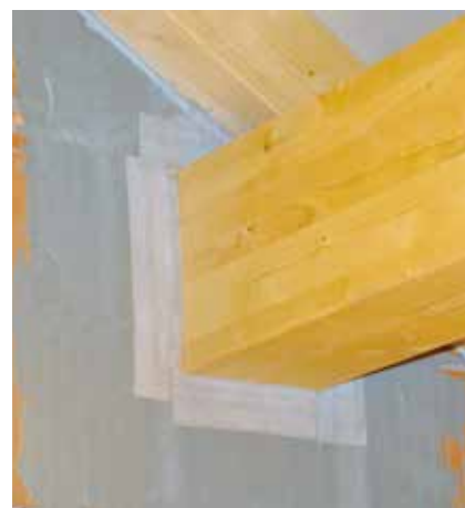
Sealing with AIR Coll 75 plaster-ready tape between wooden beam and brickwork.
