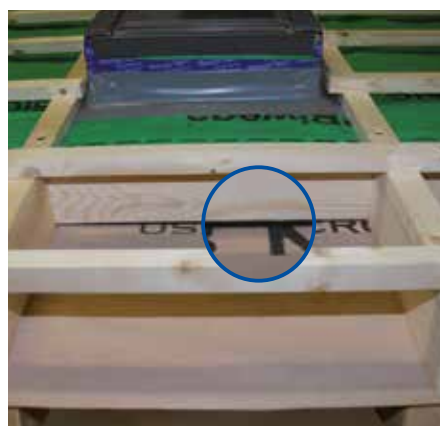
Creating an airtight seal underneath the insulation retaining frame.
