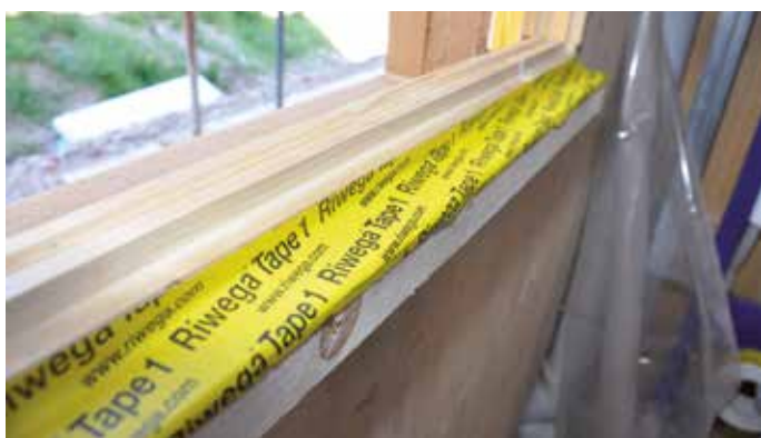
USB Tape 1 PAP X3 for sealing between the subframe and wooden wall
