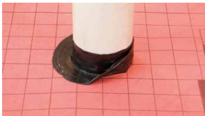
4. Model the rest of the USB Coll Flexi.
