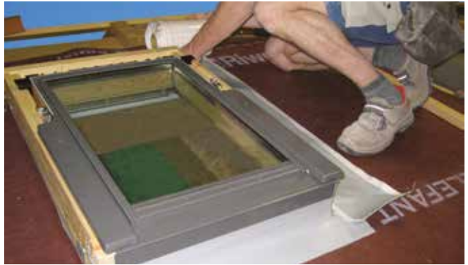
4. Apply USB Coll 150 X on both outer sides of the window
