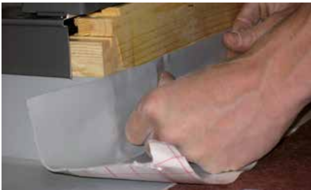
5. Lay USB Coll 150 X on the upper part of the window
