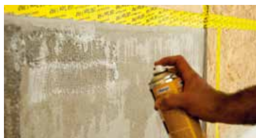
Spray head in horizontal position
