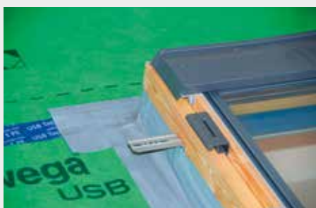
Complete sealing of a window
