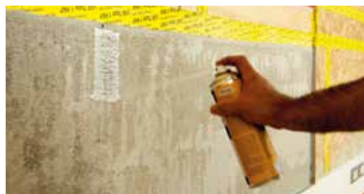
Spray head in vertical position
