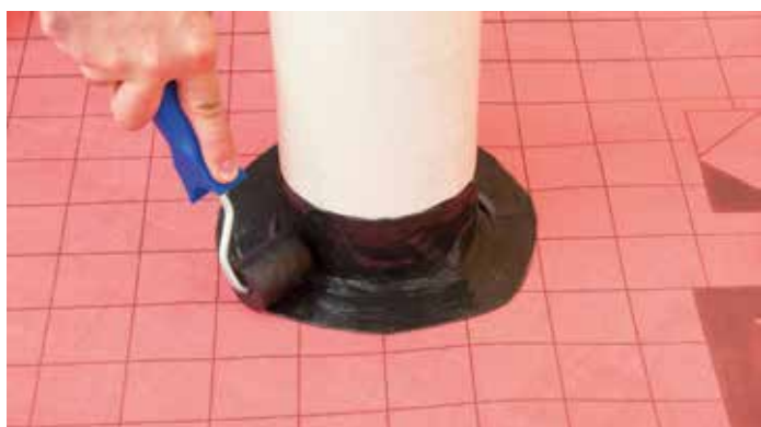
5. Press firmly onto the Riwega USB membrane with the roller.
