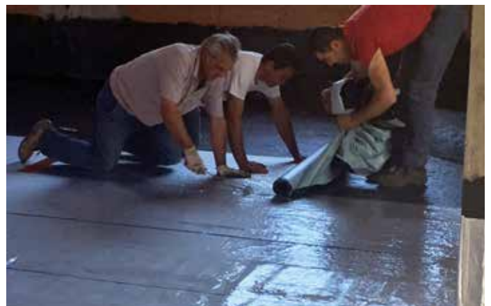
Fixing USB Coll Radon BIT barrier against radon gas
