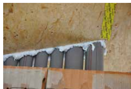
Filling of cavities, leaks and gaps in building structures
