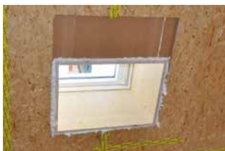
Filling leaks around the edge of a roof window
