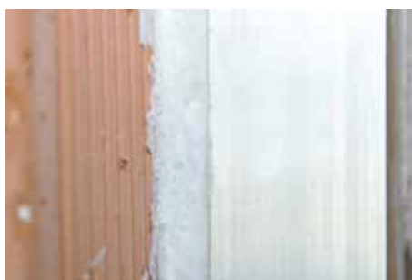
Filling between masonry and subframe
