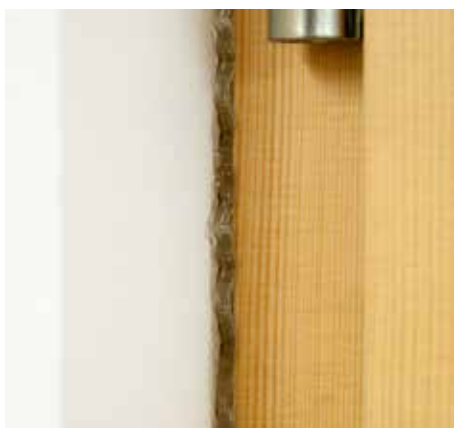
Apply USB Sil Power Fix
