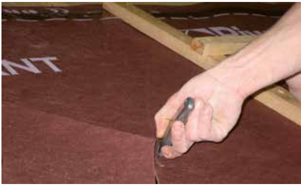
1. Cut USB Riwega breathable membrane
