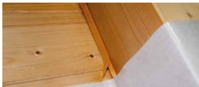
Fixing a vapour barrier to a wooden surface
