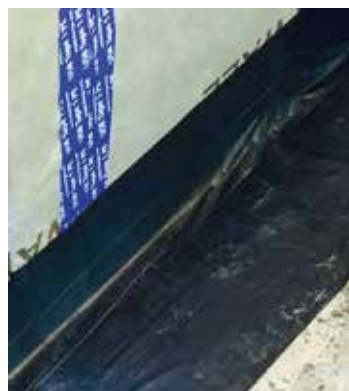
Waterproofing of X-Lam wall to floor
